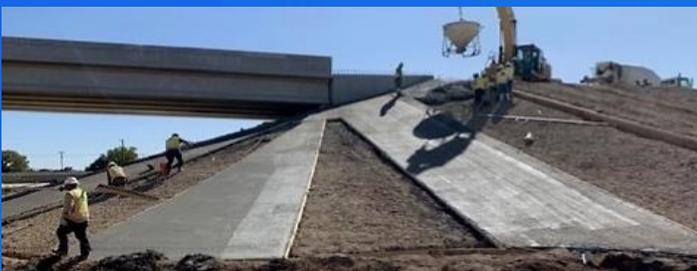
*Workers place Riprap on the north frontage road. Riprap, electrical work, and pavement markings are some of the last items needed to complete the project.*
